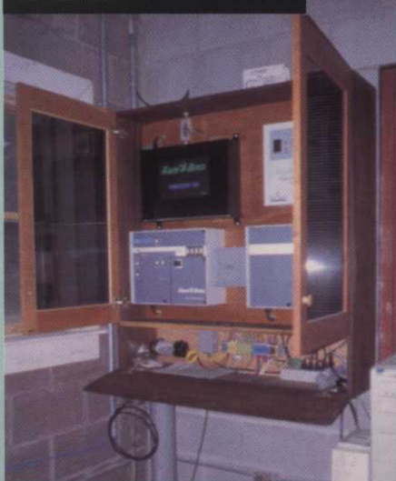
A custom built cabinet organizes irrigation control and communication components allowing for quick visual inspection and providing protection against unwanted tampering or mishandling. Photo by Darren Davis.
