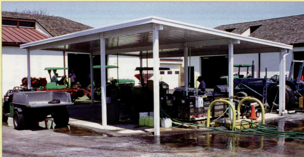
This LANDA self-contained washdown and recovery system collects and separates clippings and rinsate from golf course equipment. It also serves as a mix and load site.
