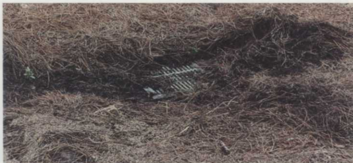
A drain basin in a depression in a pine straw area will get clogged by the moving pine straw. Photo by Joel Jackson.
