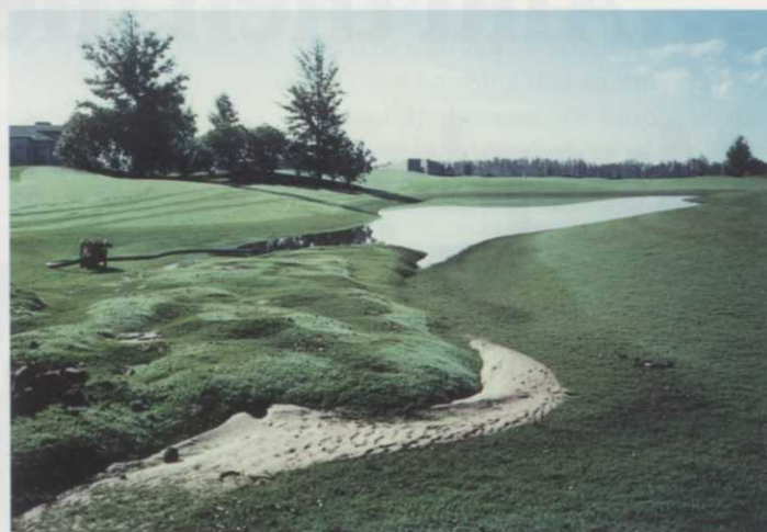
An irrigation blowout. Usually an overnight occurrence that greets you in the morning with a flood, a mound or a hole and lost irrigation coverage to deal with. Photo by Joel Jackson.
