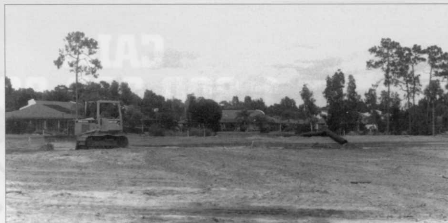
Big noise — The roar, thump and clank of heavy construction equipment has been a summer-long constant on The Forest's rebuilt Bobcat course. Looking back toward the tee, the fairway on No. 16 has been recontoured, its drainage improved. Photo by Bill Kilpatrick.
