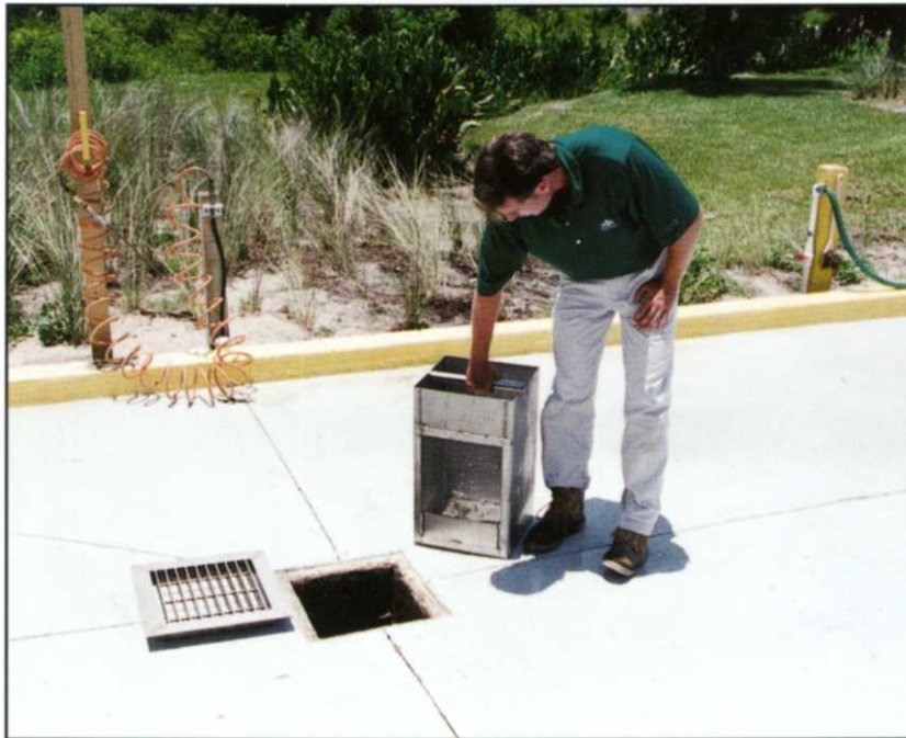
One of three removable sumps on the wash pad
