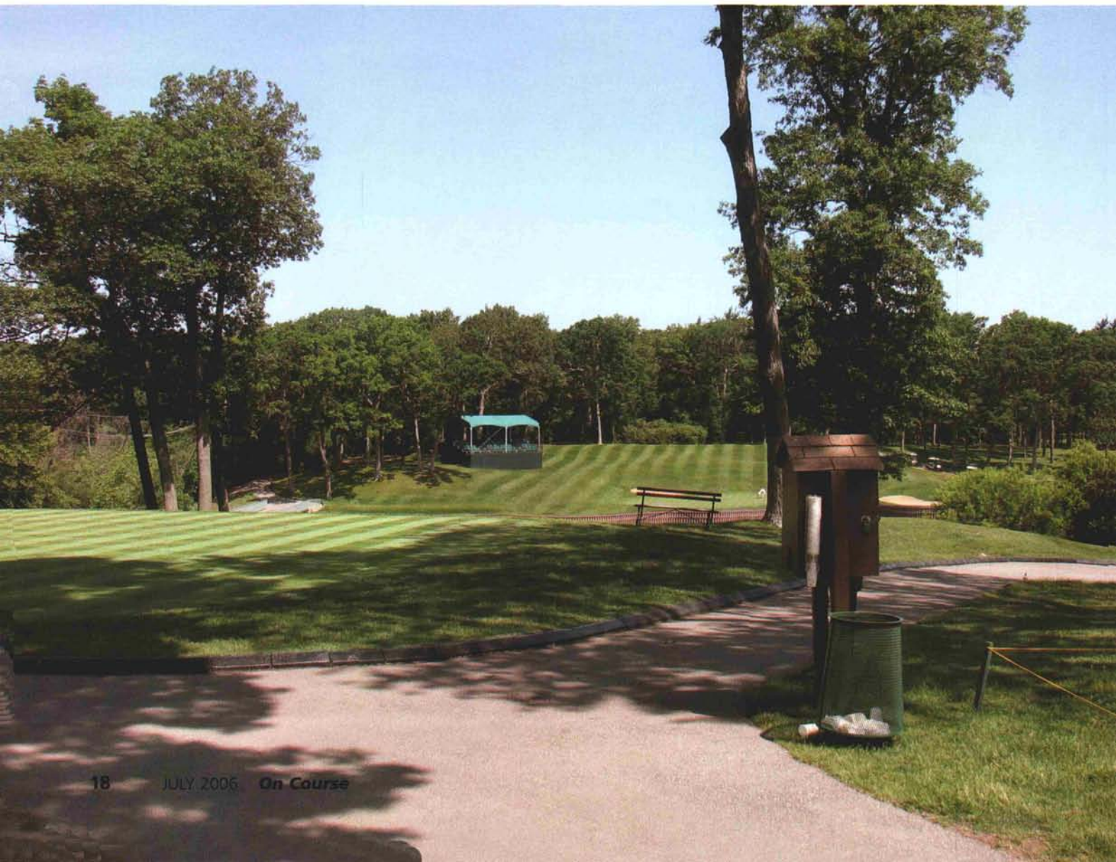
One of the many grandstands and hospitality tents being constructed in ready for the Championship.
