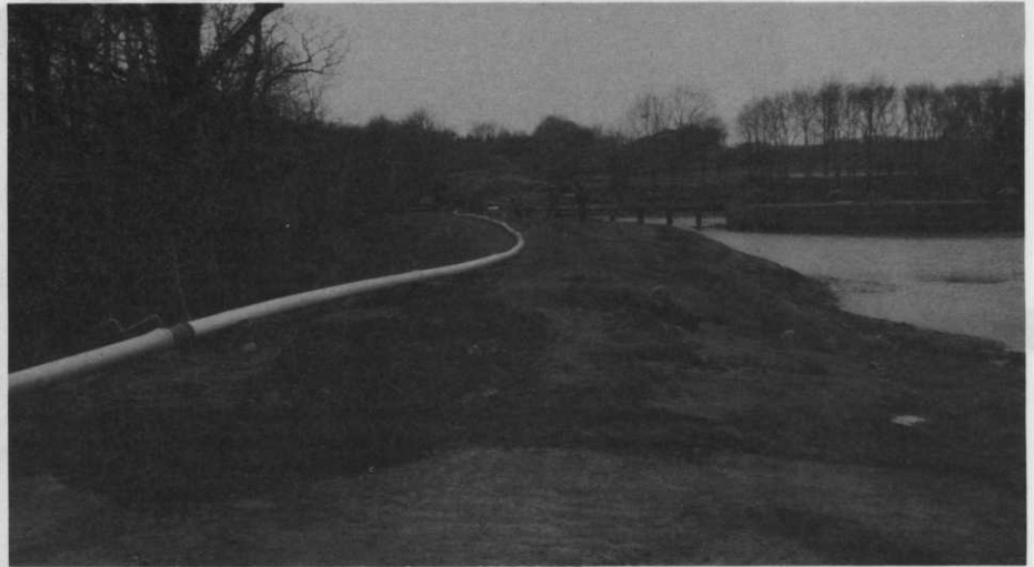
Drainage Piping. The 7th at Round Hill.
