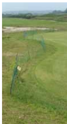
Surrounds and bunker yet to complete
