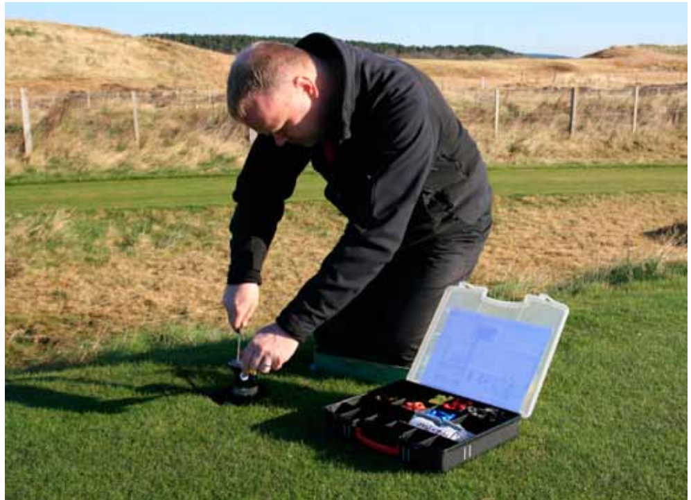
ABOVE: Sprinkler maintenance and servicing
