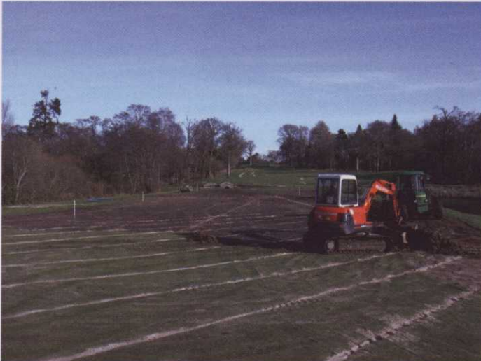
The squad is around 40% through the drainage project
