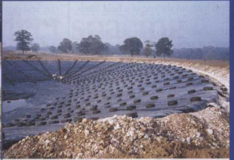
Eyhurst Golf Club: Reservoir Liner (exposed)
