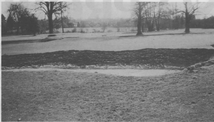
Tidy turf revetment in the face of a big bunker...
