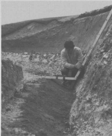
Bank shaped and base ready for first row of turf. A wooden frame was constructed to maintain the correct wall face angle.
