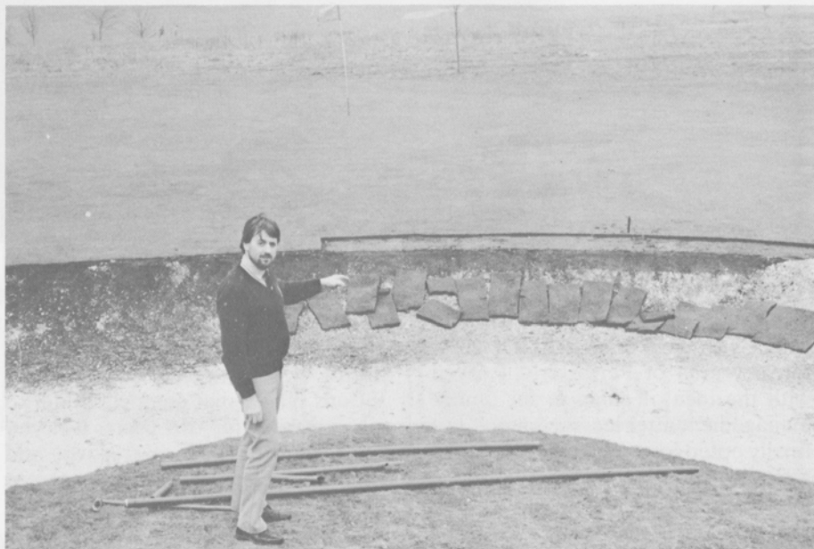
This unfinished bunker on the fringe of the Lower Course’s 12th green illustrates the MacGillivray style of trap building influenced by his training at St Andrews.
