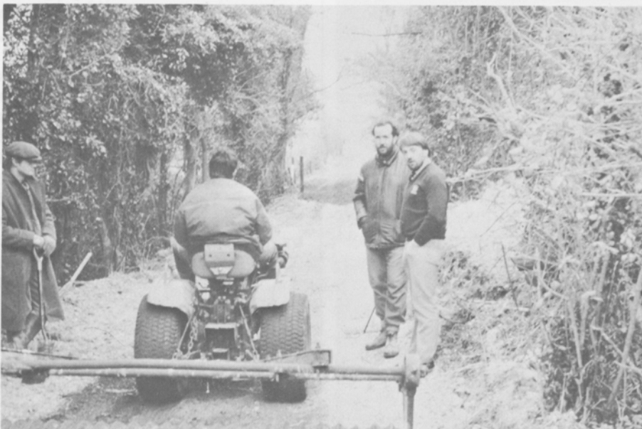
Resurfacing work to a public bridle path...
