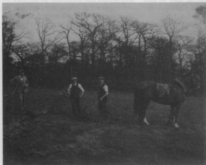
In a reservoir field, turf is being stripped prior to cultivation. The photo, taken in 1930 before the St Ives course was constructed, shows the board's founder Norman Hackett (left).
