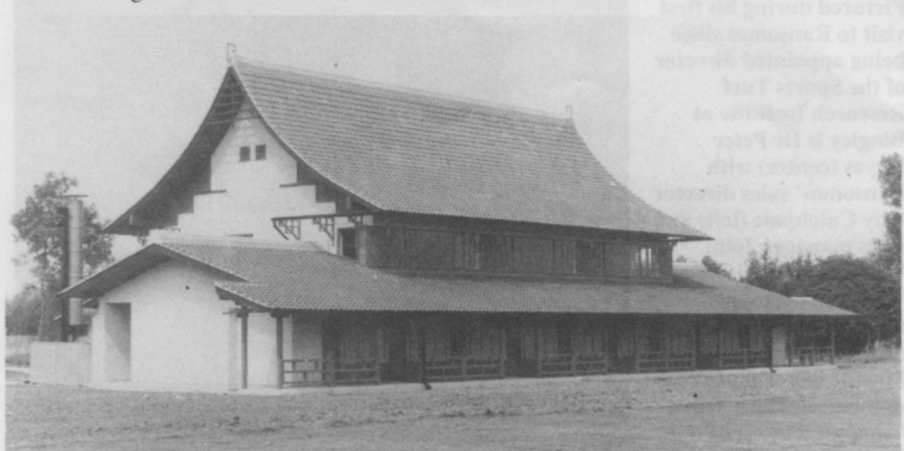
Part of the IOG's impressive new headquarters.
