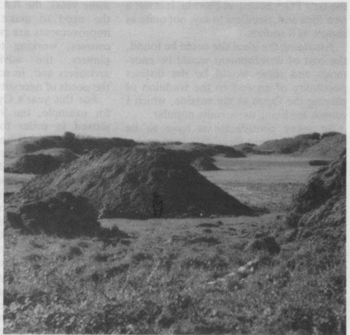
Work on the 6th fairway at Royal Birkdale.
