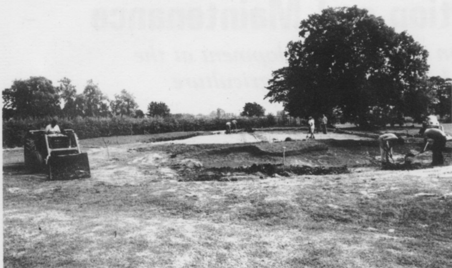
General view during the construction of the porous layer green.
