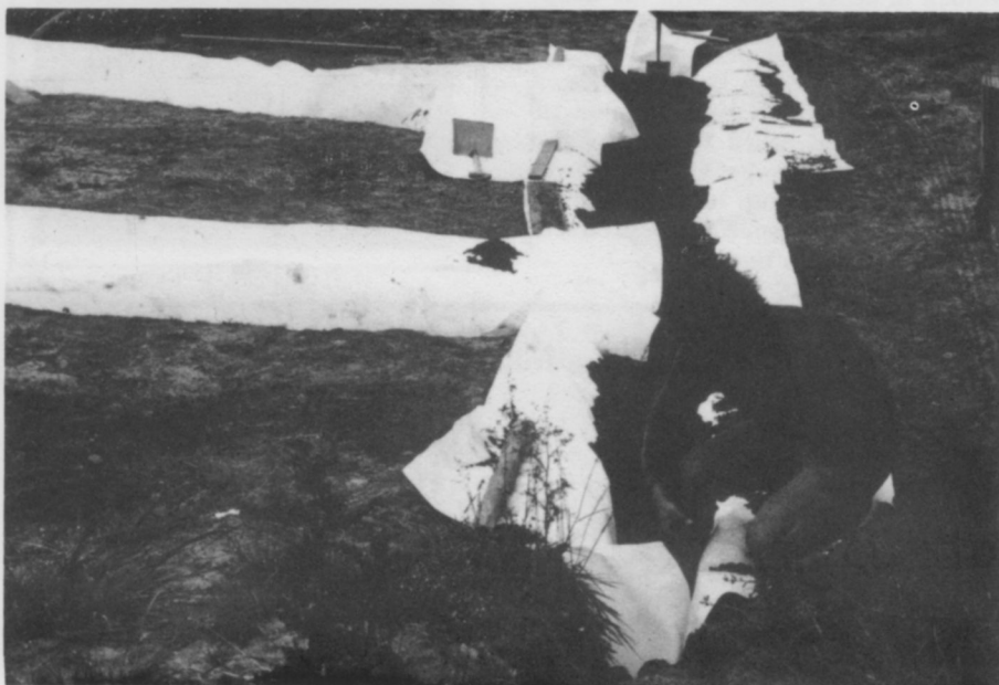
"Terram" being used as a filter membrane in drainage trenches.
