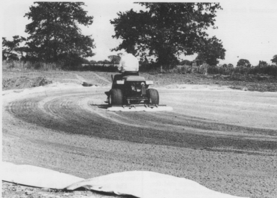
A ransomes "motor rake" being used for seedbed preparation of the "Cellsystem".
