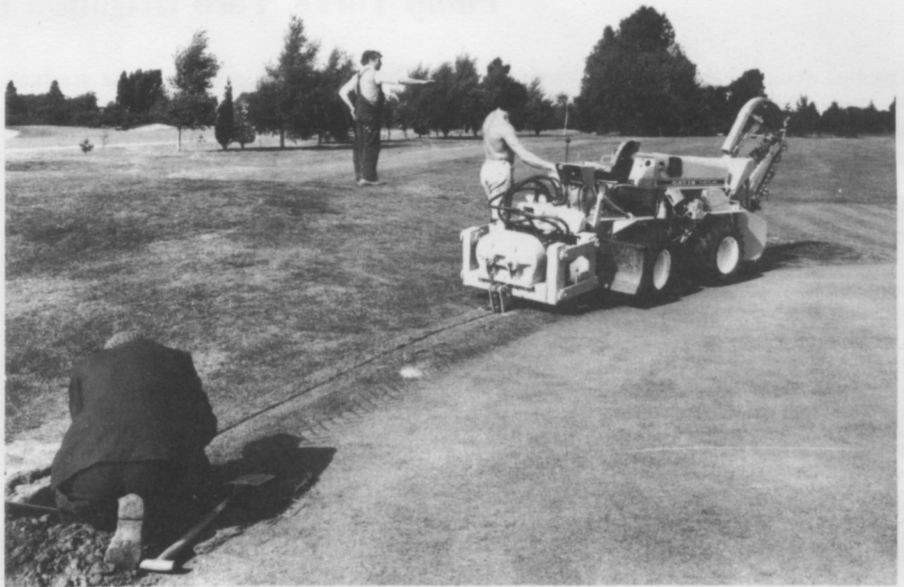
Davis Vibratory Plow working on a Midland golf course pulling in 2 in diameter plastic pipe at a depth of about 18 in around the green for the installation of pop-up sprinklers.
