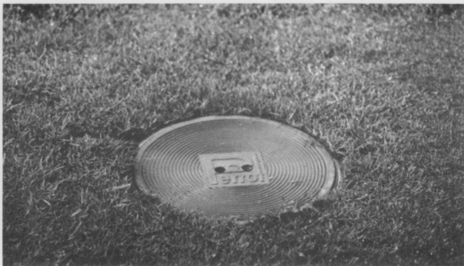
Perrot Pop-up sprinkler LVZEW, 7mm nozzle, installed at Stockport, Cheshire.
