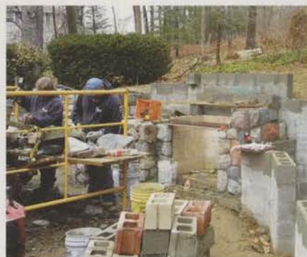
1. Fieldstone was split by hand on site for the pizza oven and fireplace. The surrounding walls and kitchen area were faced with a natural stone veneer, which was mortared onto the concrete block.
