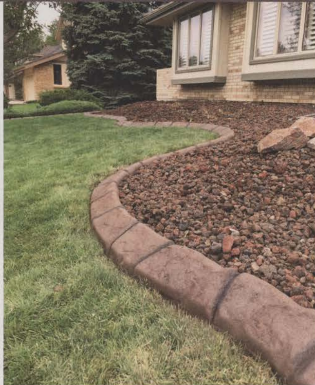
A properly installed curb can prevent mulch or rocks from washing away.
