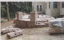
An inch of bedding sand and concrete pavers are then installed and cut to fit the patio area.
