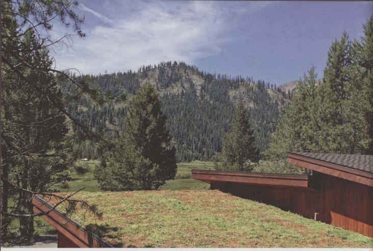
Green roofs, or living roofs, are gaining popularity as a method of beautification and storm water filtration on new and existing structures.
