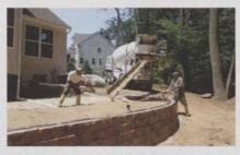
A ready-mix concrete truck delivers flowable fill, a mix of sand, cement and water that reduces the longer installation time using dense-graded
