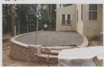
Once the flowable fill is poured in lifts and each allowed to harden, a 4-in. thick compacted aggregate base is installed.
