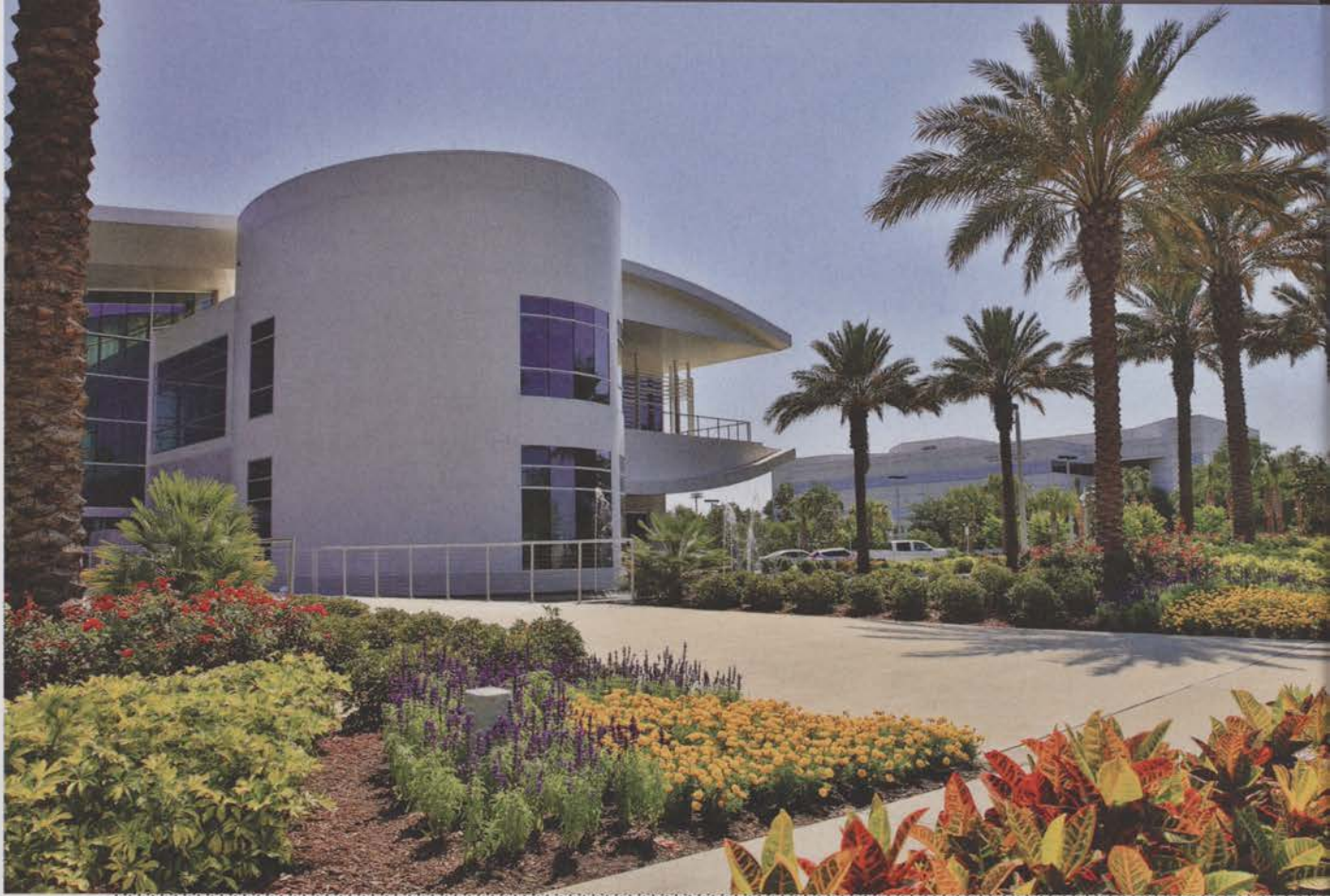
ABOVE: The company's landscape installation work at Jim W. Henderson Administration and Welcome Center at Embry-Riddle Aeronautical University in Daytona Beach, Florida, was completed in 2013.
