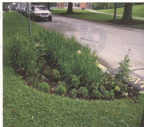
A rain garden will collect contaminants that run off of asphalt and from the roof. It should only be able to hold water temporarily while it absorbs during storms, and then it filters through the amendments of the soil layers.
