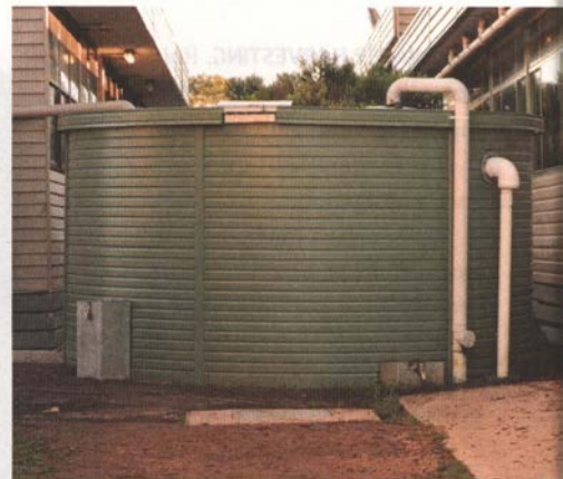
Rainwater can be collected from rooftops or other above-ground hard surfaces. It then goes through a pre-filter and is piped into the containment system.
