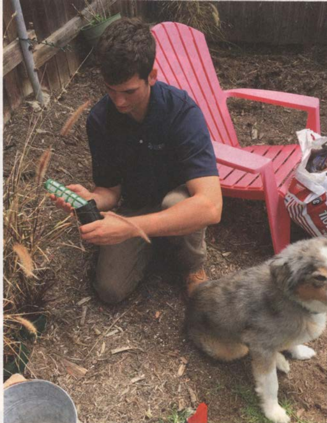
Gabriel D. Michael, Blue Watchdog's director of operations, joined by the company mascot, Wallace, inspects a filter. Owner Patrick Crais says filters should be cleaned every year and can last between two and five years.
