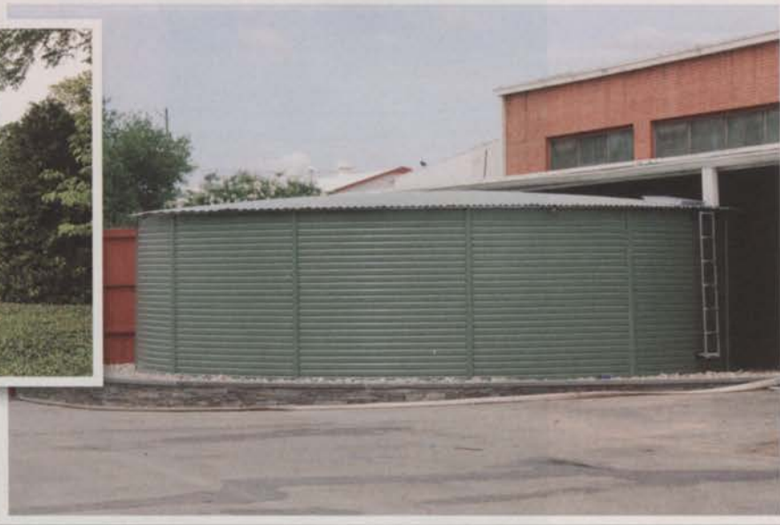
Above: One of Lambert's residential cistern installations holds 46,000 gallons of water underground. Right: Lambert Landscape Co. installed a 20,000-gallon cistern to catch rain off the company's roof.
