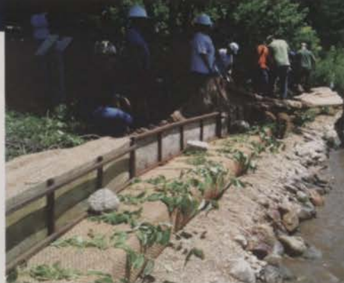
Shoreline remediation makes sense for many landscape contractors.
