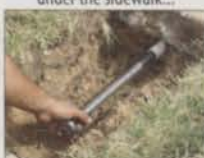
Remove Sidewalk Sleever from the sleeve.
