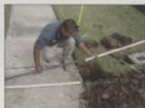
Place a sleeve on the Sidewalk Sleever.
