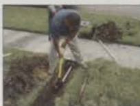
Hammer tool w/sleeve under the sidewalk...
