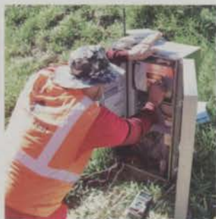
New technology makes systems more efficient.
