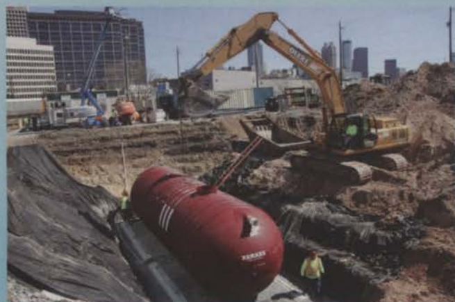
Most below ground cisterns can be buried deep enough so that the water level in the tank is below the frost line.
