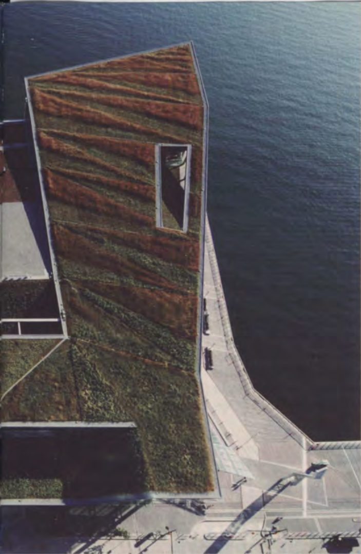
The North American green roof industry grew 28.5 percent in 2010, according to Green Roofs for Healthy Cities annual survey. The extensive green roof (above) on the Vancouver Convention Centre won a 2010 Award of Excellence from GRHC.
