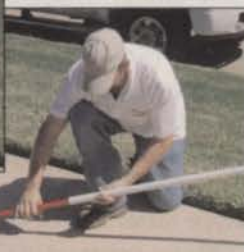
Place Sidewalk Sleever inside pipe
