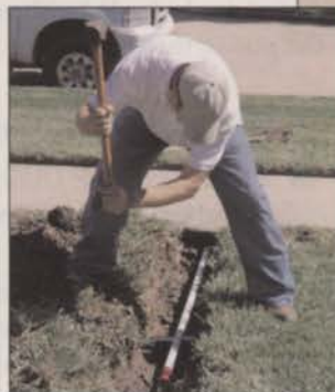
Hammer Sidewalk Sleever & pipe under obstacle
