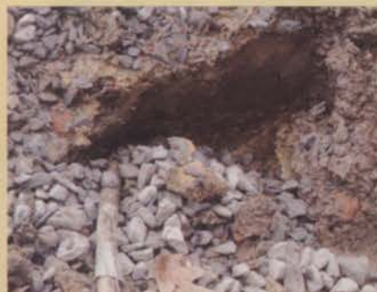
Underground irrigation lines can be damaged by an unaware contractor.
