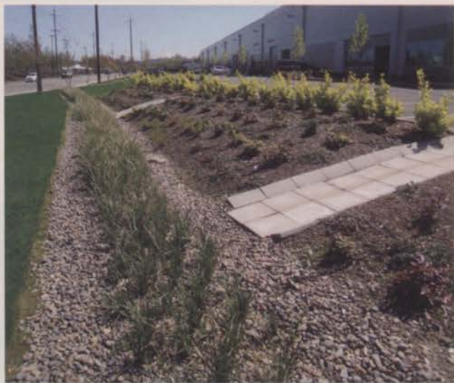
At left, an array of solar panels power the company's offices. Below, a bioswale – an installation designed to filter storm runoff – the firm installed and maintains for a commercial client.
