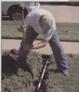
Hammer Sidewalk Sleeve & pipe under obstacle
