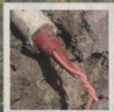
Pull wires back through the installed pipe
