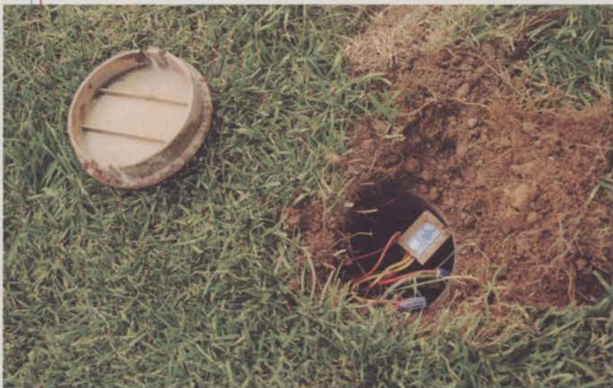
Water-proof field decoders are attached to each valve solenoid in a two-wire system. Field decoders have unique station addresses and receive program signals from the controller, activating the sprinklers in that zone.
