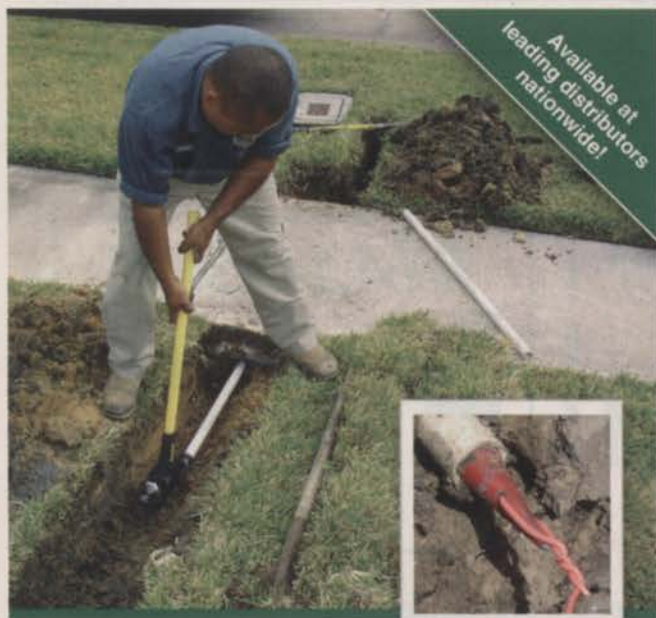
Pull wires back through the installed pipe
