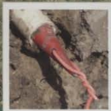
Pull wires back through the installed pipe
