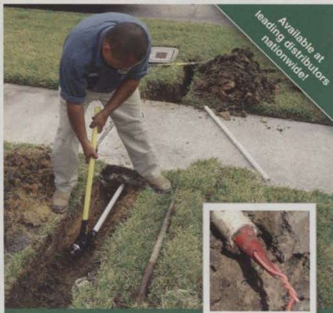
Pull wires back through the installed pipe
