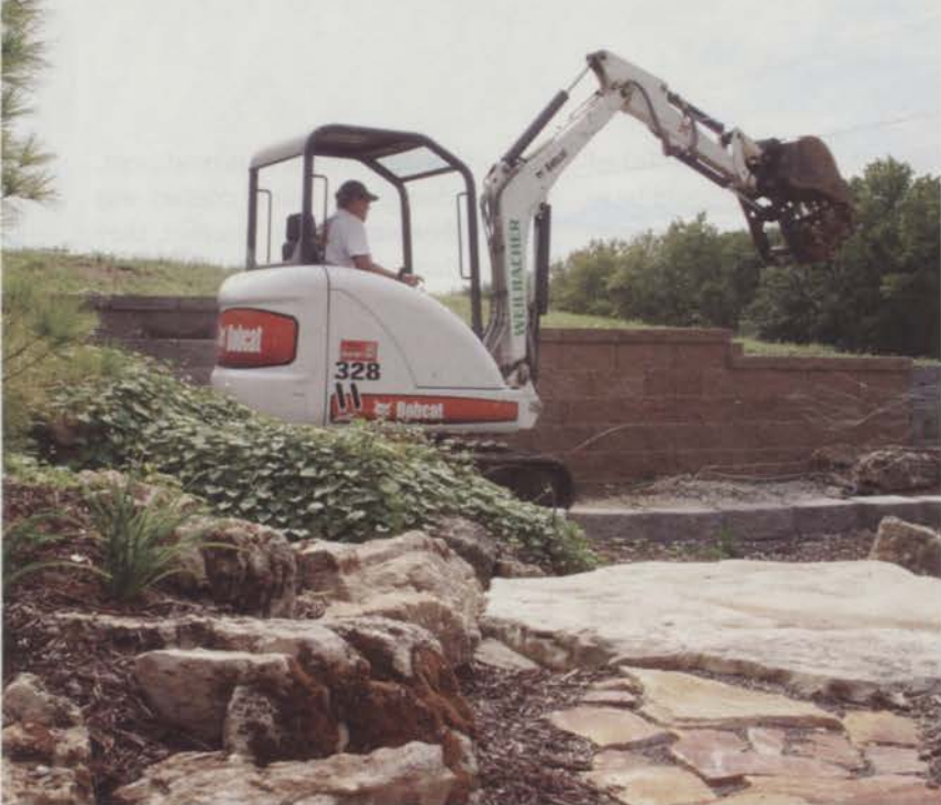
Weilbacher Landscaping uses its Bobcat 328 compact excavator for the hardscapes and water features it installs.
