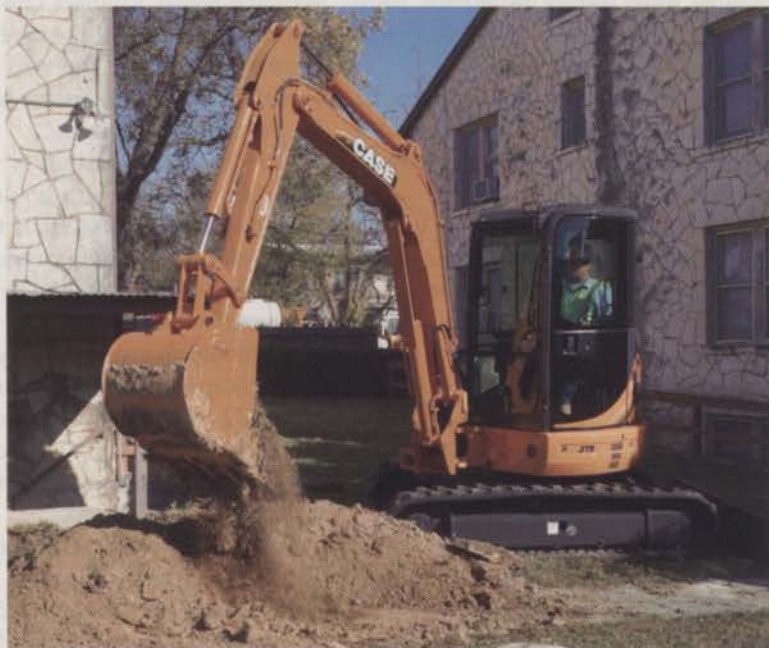
Outdoor Environments crews use a mini excavator 50 percent of the time. On dusty sites, keeping the machine greased is important.
