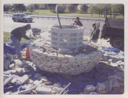
The biggest challenge of the project was building the structure of the original concept. The basin was excavated to a depth of 3 feet with a 15-foot circumference. The backbone of the Preserve became a 4-by-4-foot drywell, which was lowered into place with a backhoe on a high-traffic roadway. Once the drywell was secured, each piece of South Bay Quartzite was milled and cemented
