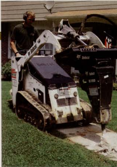
There are many reasons landscape contractors have been opting for smaller construction equipment, including accessing tighter areas and getting work done at faster speeds with less labor. Photo: Bobcat
