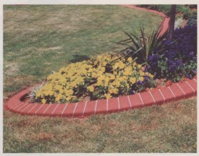
Concrete sealer, similar to what contractors apply over stamped concrete patios, is required to ensure a curb's longevity. As his customers' curbs age, Retzlaff plans to add a maintenance service that includes pressure washing curbs and reapplying sealer.
