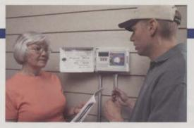
water. The non-volatile memory feature stores a system's program indefinitely, acting as insurance against problems like power outages. Controllers also come remote-control ready to allow contractors to manage a system off site.
