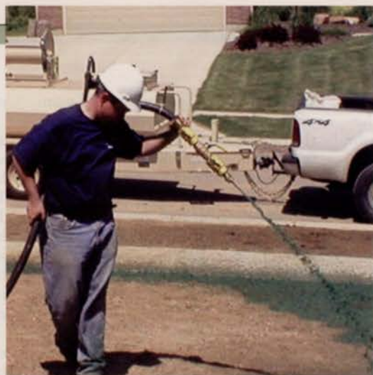
Contractors and manufacturers agree that most hydroseeding jobs can be done by one contractor with one machine in one step. Photo: Finn Corp.
