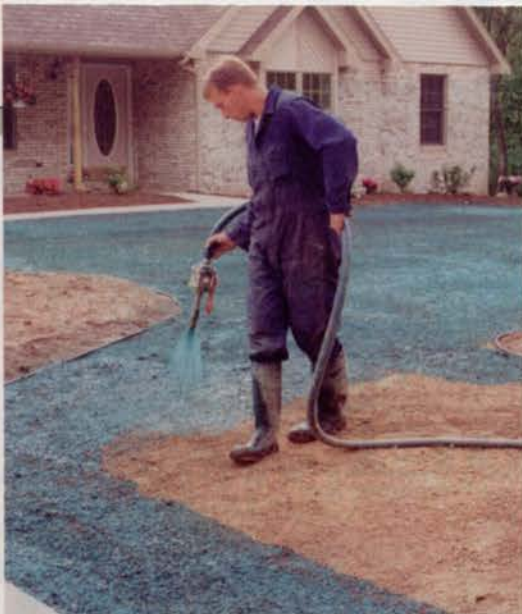
The dyed mulch used to hydroseed helps contractors see where they have sprayed to ensure an even application. Photo: Turbo Technologies
