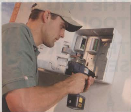
A contractor installs a controller for a residential irrigation system. Photo: Rain Bird
