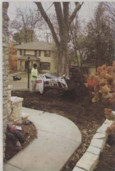
Compact loaders allow efficient movement through tight work areas. Photo: Bobcat
