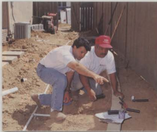
Landscape contractors install irrigation piping on a jobsite. Photo: Hunter Industries
