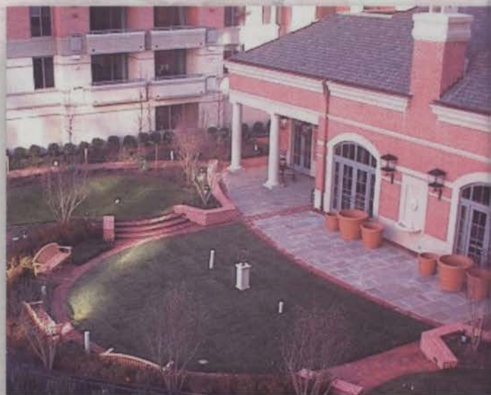
An example of a "green roof," installed by Bozzuto Landscape Co., that is becoming popular atop commercial buildings, according to an IFMA research study. Photo: Bozzuto Landscape Co.
