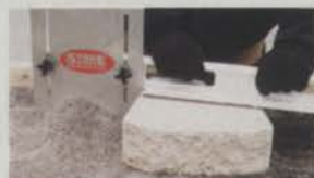
Lay main frame on stone and push grade blade into base material
