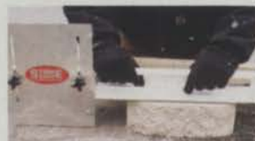
Push or pull main frame across stone leveling base material with blade
