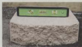
Ensure that the first stone is level
