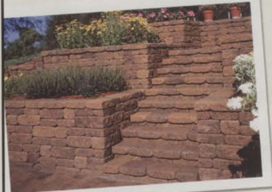
Private Residence, Scandia, Minnesota, in VERSA-LOK Weathered Mosaic
