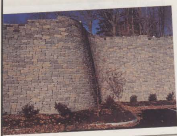
Municipal Parking Lot, Town of Wilton, Maine, in VERSA-LOK Weathered Mosaic
