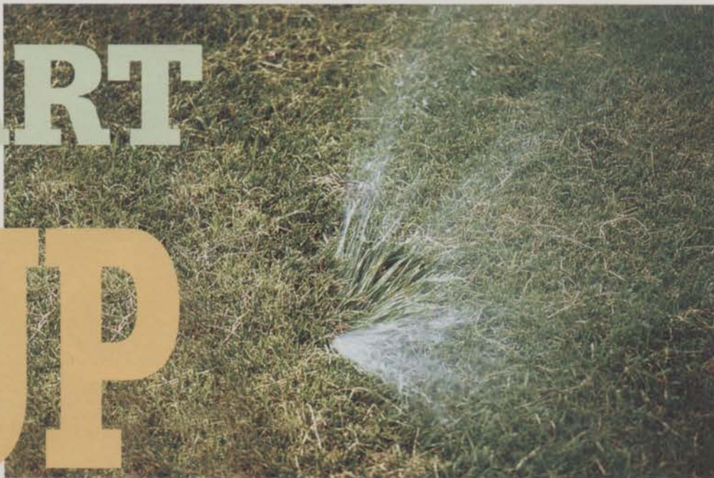
Adjusting the height on pop-up sprinkler heads as a regular part of irrigation system start-up and maintenance can help eliminate the chance of a stifled spray like the one pictured above.
