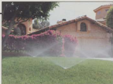
Because of their shorter radii, spray heads are best used in smaller areas like home lawns.
