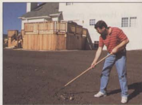
Regardless of which method a contractor chooses when installing a lawn, soil preparation is a must. The site should be cleared, graded, inspected and treated with a lawn roller. Photo: Turfgrass Producers International
