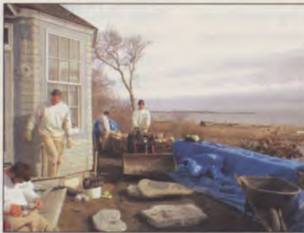
Instead of moving large boulders with shovels, Maffei Landscaping Contractors' crews use the Dingo compact utility loader to simplify the job. Photos: Maffei Landscaping Contractors
